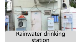
Rainwater drinking station
