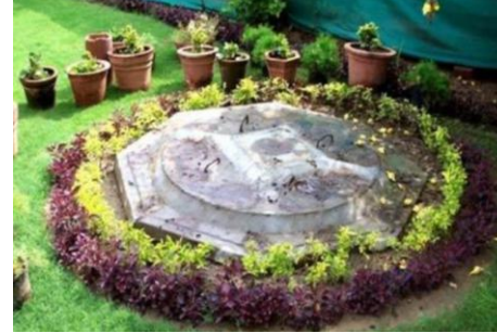
Parikh House – A resident of Ahmedabad city : Rainwater harvesting systems along ground water recharge structure (recharging existing bore well); water used for drinking purpose
