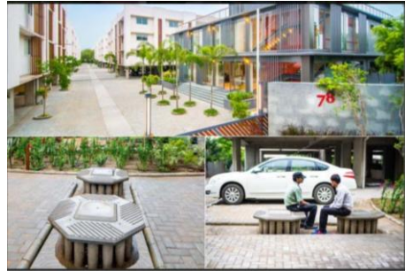
78@Gokuldham, Residential society, Ahmedabad : Rainwater harvesting systems developed in alignment with storm water management system
